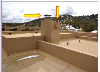
3. Chimney present with clay flue, spark arrestor and rain cap with a second gasfired exhaust jacket are in **Satisfactory Condition**.
