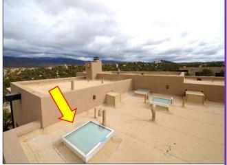
Torch-down roof membrane was professional installed surrounded by Parapets and Velux Skylights are in Satisfactory Condition.
