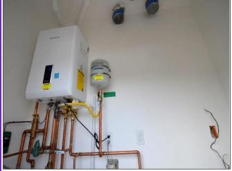
13. Southside Mechanical Closet for the **Navien** Boiler & Domestic H<sub>2</sub>O, was professional installed and is in **Satisfactory Condition**,
