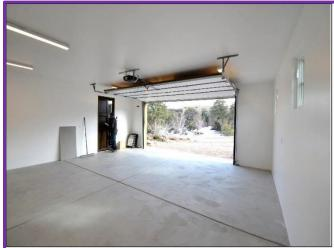
19. Garage with concrete floors and fully painted 5/8" drywall as per code and automatic overhead garage door are in **Satisfactory Condition**,
