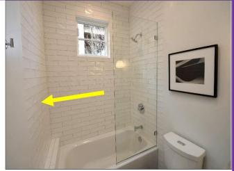
32. Tempered glass panel for the Bathtub is backwards and should be installed at the other end to properly access the faucet as per UBC & State CID Codes.
