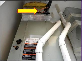
10. **Trane** Furnace and AC Unit has not been completely hooked-up with the refrigerated pipes.
