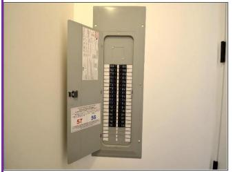
21. 2nd **200Amp** electrical Subpanel inside the Laundry Room is in **Satisfactory Condition**,
