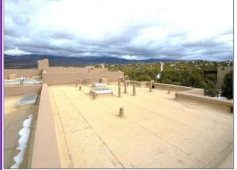
Torch-down roof membrane was professional installed, and maintenance should occur every 3years and roof is in Satisfactory Condition,
