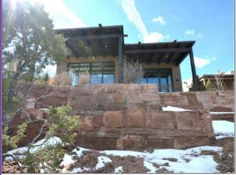
39. Eastside view of House perched on massive retaining rock walls that are stepped-back with terraces and weep drainage
