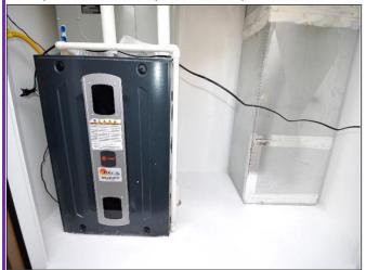
Northside Mechanical Closet with **Trane** Furnace and AC Unit was professional installed and is in **Satisfactory Condition**, except for, see picture #10.
